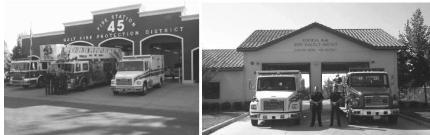
FIGURE 6.6 Station #45 and Station #46
