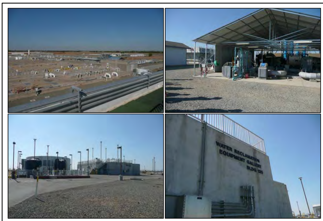
Figure 3.1-2: Existing Facilities at SRWTP
