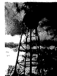
Elevated Storage Tank
